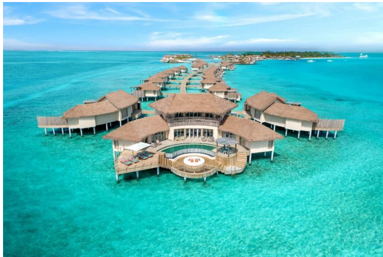
ABOVE: AERIAL VIEW OF THE THREE-BEDROOM OVERWATER RESIDENCE
